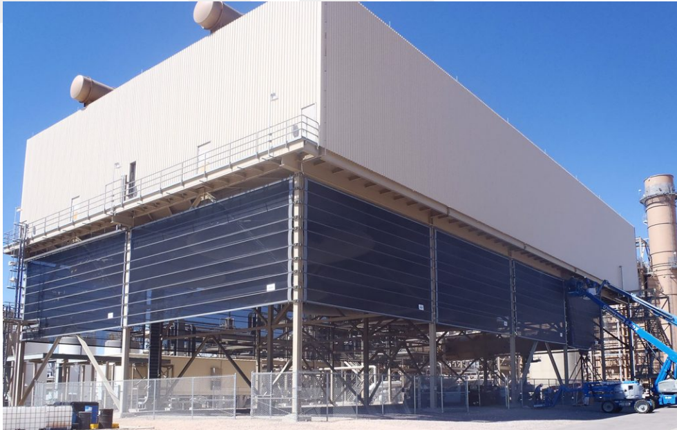
Figure 3: Gale breakers deployed (Source: galebreakercooling.com )
