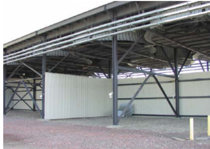
Figure 4: Cruciform walls (Source: Maulbetsch and DiFilippo)
